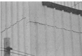
Asbestos-Cement Siding
